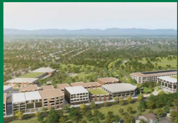
Centrala in Angeles, Pampanga
