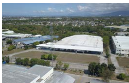
ALLHC's cold storage facility in Laguna
