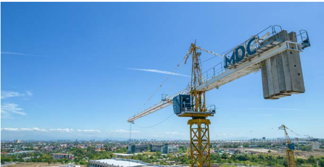
Construction was in full swing for MDC, completing 29 projects in 2022
