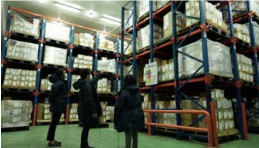
ALogis Artico has a total cold storage capacity of 10,300 pallet positions.
